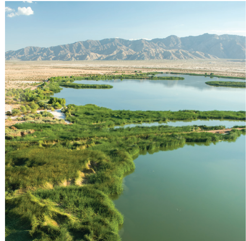
Las Arenitas Water Treatment Plant wetlands
