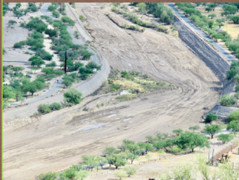
June 1, 2020 View of preserved wetland area near outfall after sediment removal
